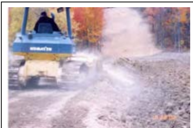
Fig. 12. Moderately dry topsoil is being replaced on the affected site now that Phase 1 deep ripping of the compressed subsoil is complete.
