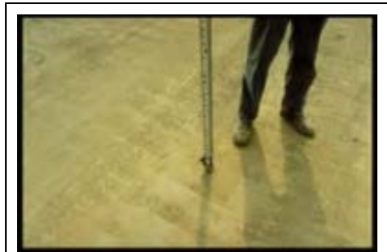
Fig. 3. Construction site with significant compaction of the deep basal till subsoil extends 24 inches below this exposed cut-and-fill work surface.
